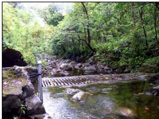
Figure 8. The intake for the Honolua stream diversion.
