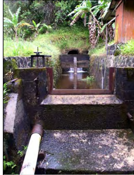
Figure 9. Water flows through the diversion and is piped back to Honolua stream.
