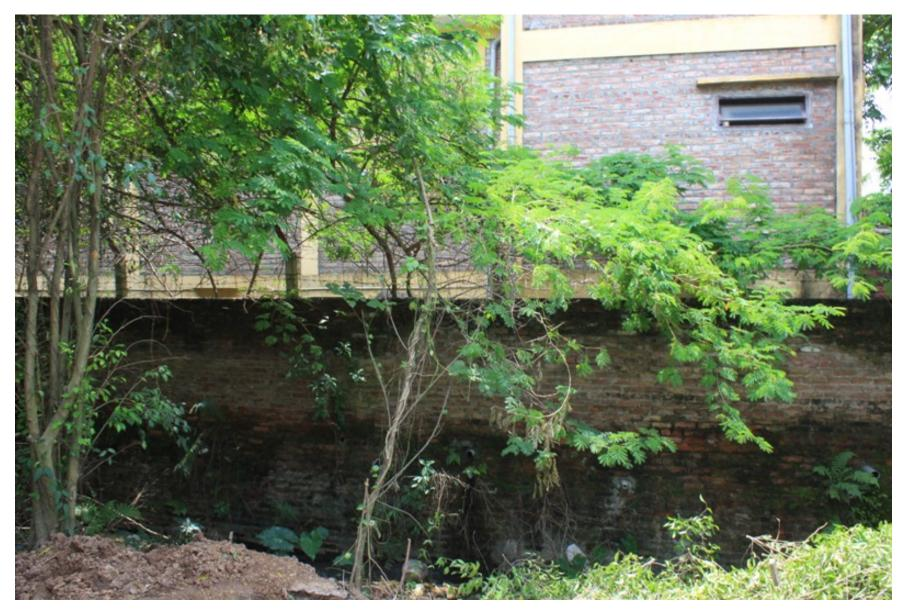
Figure 3 Dividing wall with neighbor's effluent pipes draining into open ditch on EcoPark property
